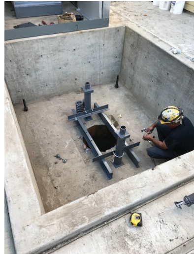
The pit is poured by use of a template and the elevator is lowered in.
