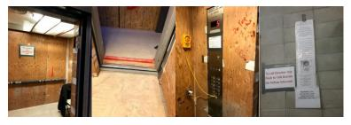
Once usage as a Construction Hoist is complete, the cab is refurbished to factory standards, or with one of numerous upgraded finish options, and the elevator receives a permanent DOSH operating permit.
