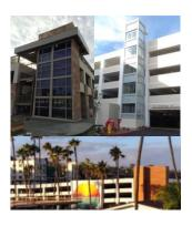
As with any elevator, it is recommended that a Modular Elevator be incorporated early in the project design process to accommodate the modular unit's footprint, any building connections and required machine room space. This leads to a smooth Building Permit process (avoiding deferred submittals), eliminates any reconfiguration of the building and provides for efficient construction.
