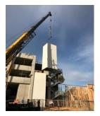
The MEM Elevator System solution vastly improves the efficiency of the construction process and offers time savings that results in costs savings to the project. This allows the Modular Elevator to be manufactured in the plant simultaneously as the construction of the Parking Structure.
